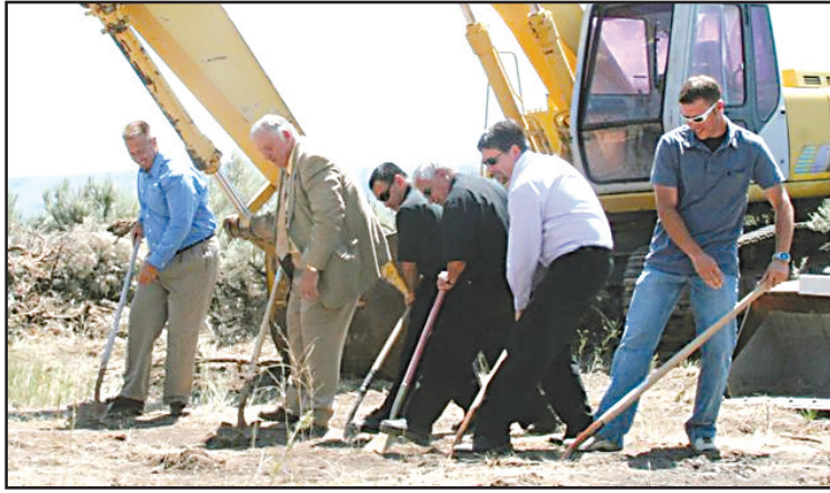
BREAKING NEW GROUND — Leaders from Holy Spirit Catholic Community and Pocatello scooped the first shovelfuls of dirt July 28 from a site near the existing parish for a new church and school. From left are Kevin Strehle from BCDM Architects; Pocatello Mayor Roger Chase; Father Adrian Vazquez, parochial vicar; Father Enrique Terriquez, pastor; Mark Dahlquist, Building Core Committee chairman; and civil engineer Jeremy Manska. (ICR photo courtesy of Holy Spirit Catholic Community)
